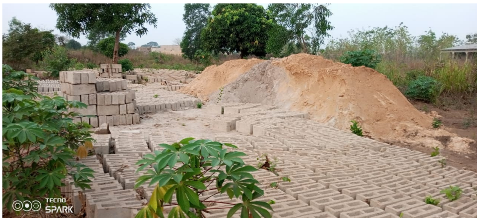
Cement blocks for the church building at Rock BC
