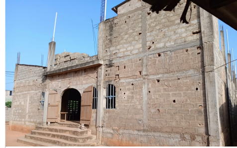
Conqueror BC, building ready for the concrete
