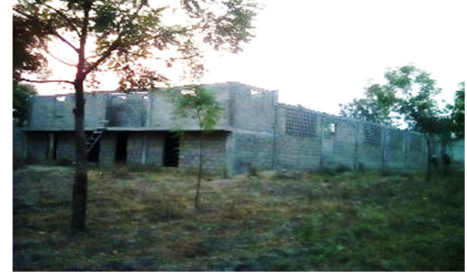
Construction Progress at FBT
