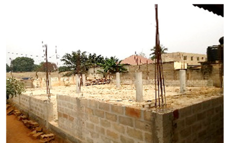
Construction Progress at GSBC
