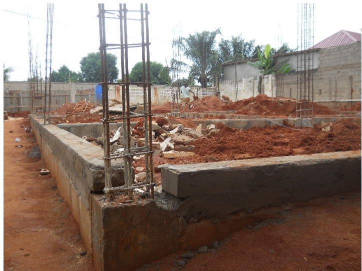
Temple foundation work
