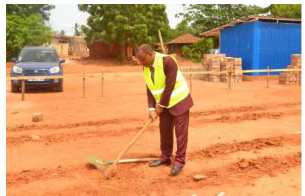
David making the first diggings on the launching day.
