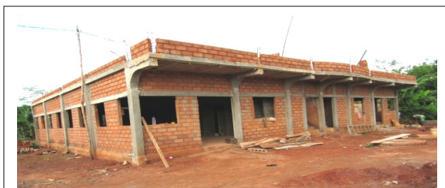
Orphanage dorms construction progress
