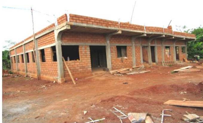
Orphanage in Togo nearing completion!
