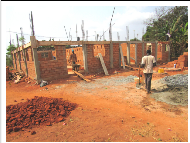
The orphanage dorms in construction
