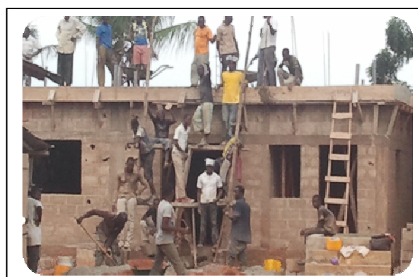
The brethren at work for the concrete: 09/26/2014
